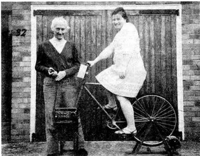
G3TWS and wife G8TWS testing a pedal-powered generator developed by John for use in Zaire to power an hf network linking mission hospitals
